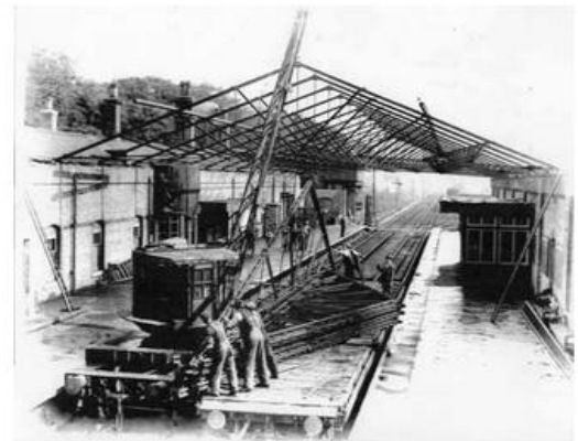
Removal of station roof in 1941
