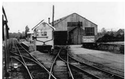
View of the signal box from the train (1970) (King)
